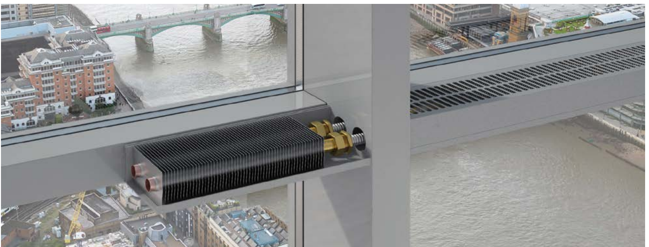
An example of installation without fixing supply and return pipes, passing through the facade.
