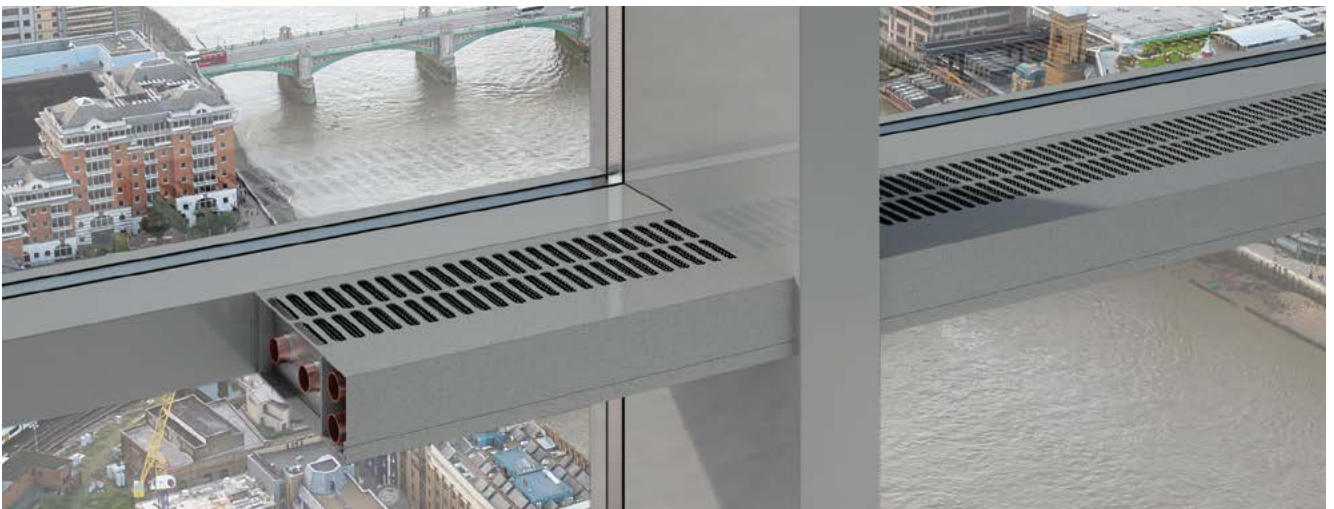
An example of installation passing through the facade, with fixing the supply and return pipes
