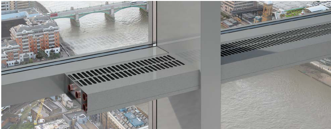
An installation passing through the facade, with fixed supply and return pipes.
